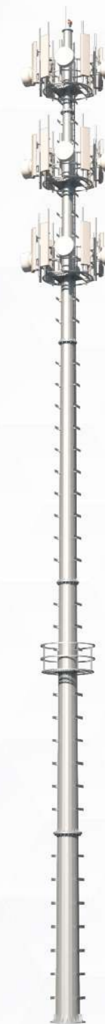
Telecommunication Monopole p104
